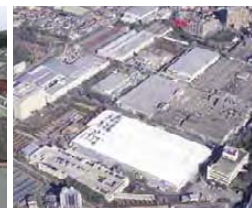
NSK Fujisawa Plant
