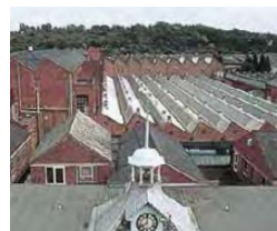
NSK Newark Plant
